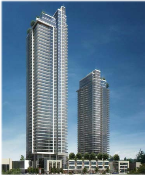
Image credit: Anthem Properties / Chris Dikeakos Architects
