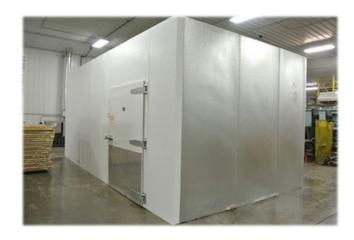
It is impractical to comply with the acceptable solution and install thermal protection in the interior of a cooler or freezer. Gypsum board, for example, will deteriorate over time due to the cold, damp environment and does not lend itself to easy cleaning to the extent that may be required in the cooler and freezer.
