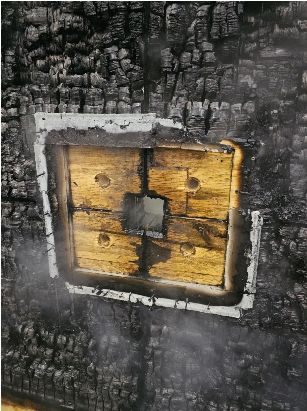
Figure 13. Fire side at HSS steel column penetration with steel plate removed.
