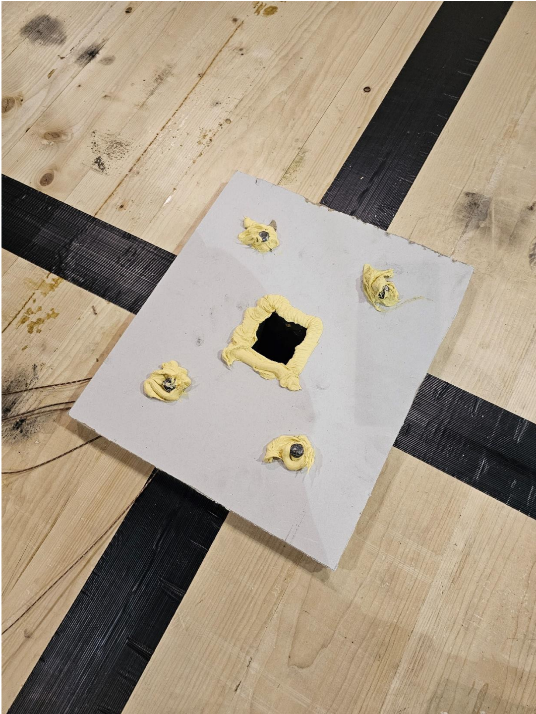
Figure 7: Unexposed Side Steel Plate Connection Finished with Gypsum Board and Fire Caulking
