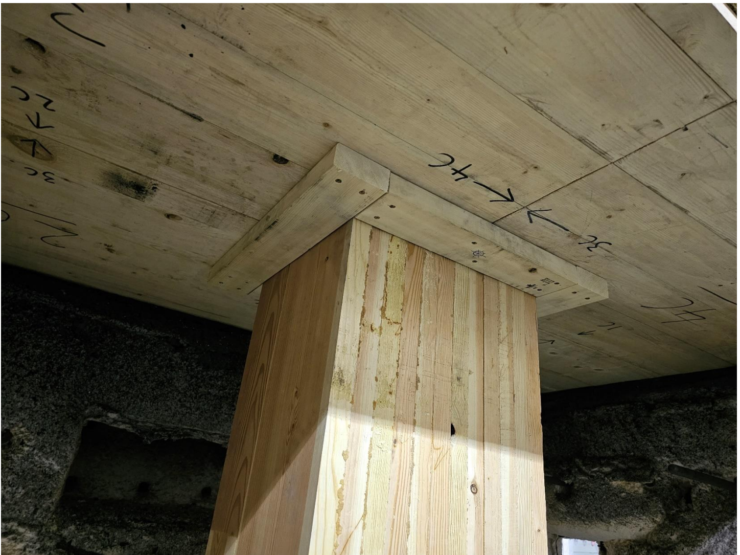
Figure 8: First layer of wood protection around steel support
