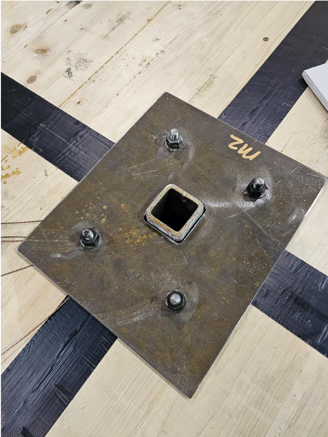
Figure 6: Unexposed CLT surface after plate installation.
