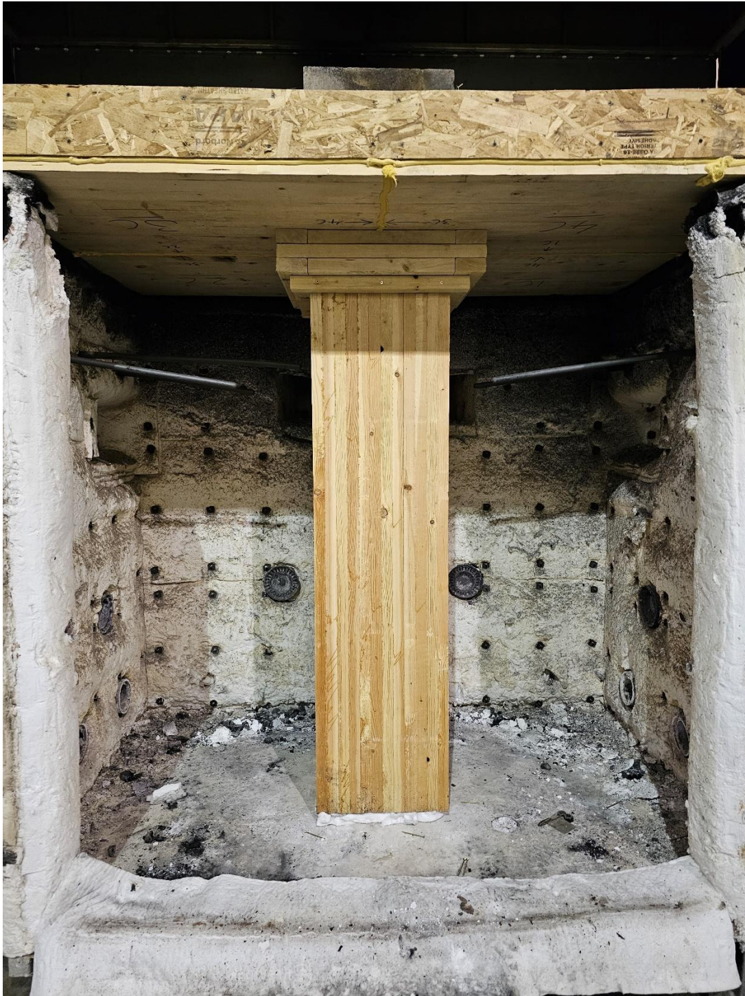
Figure 5: Exposed side of the test assembly prior to the fire test.
