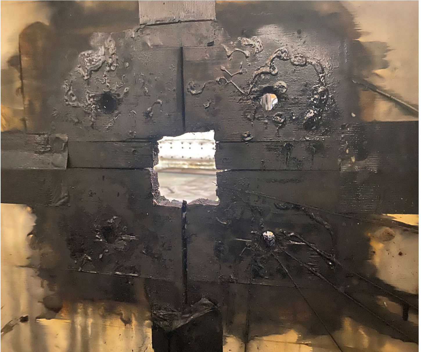
Figure 13. Non-Fire side at steel column 3 inch x 3 inch steel column penetration with steel plate removed.
