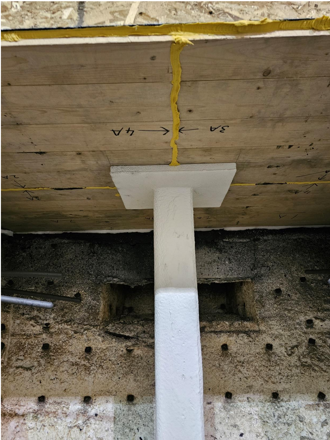
Figure 8. CLT with Intumescent Painted HSS Steel Column Prior to Testing
