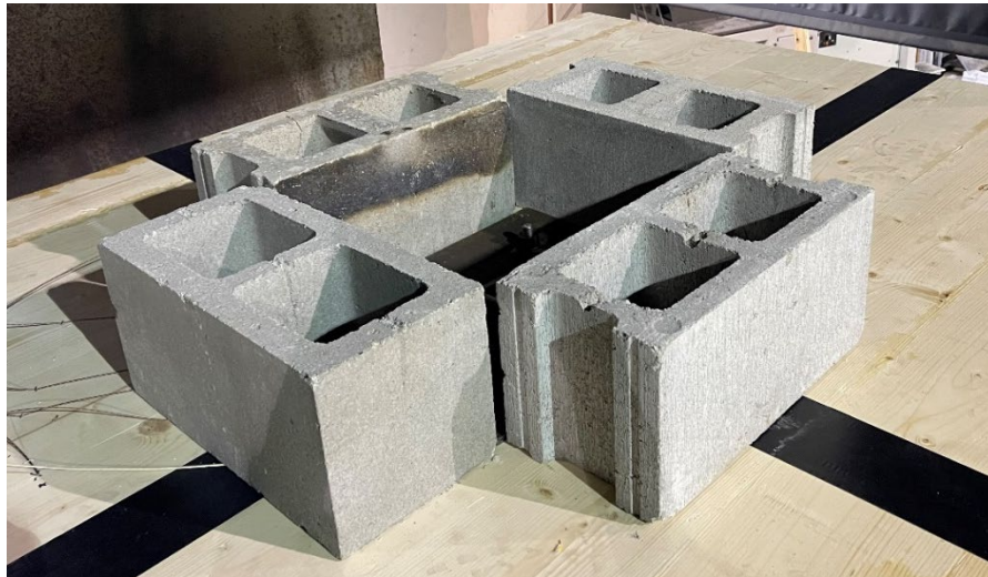
Figure 1. Concrete blocks on top of panel
