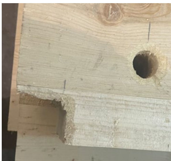
Figure 4. Photos of the panel edge after field fabrication by trades
