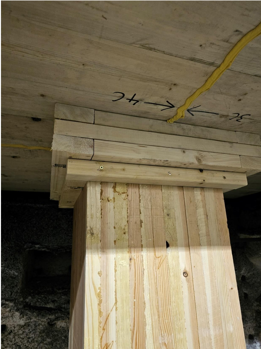
Figure 9: All layers of wood support around steel support.
