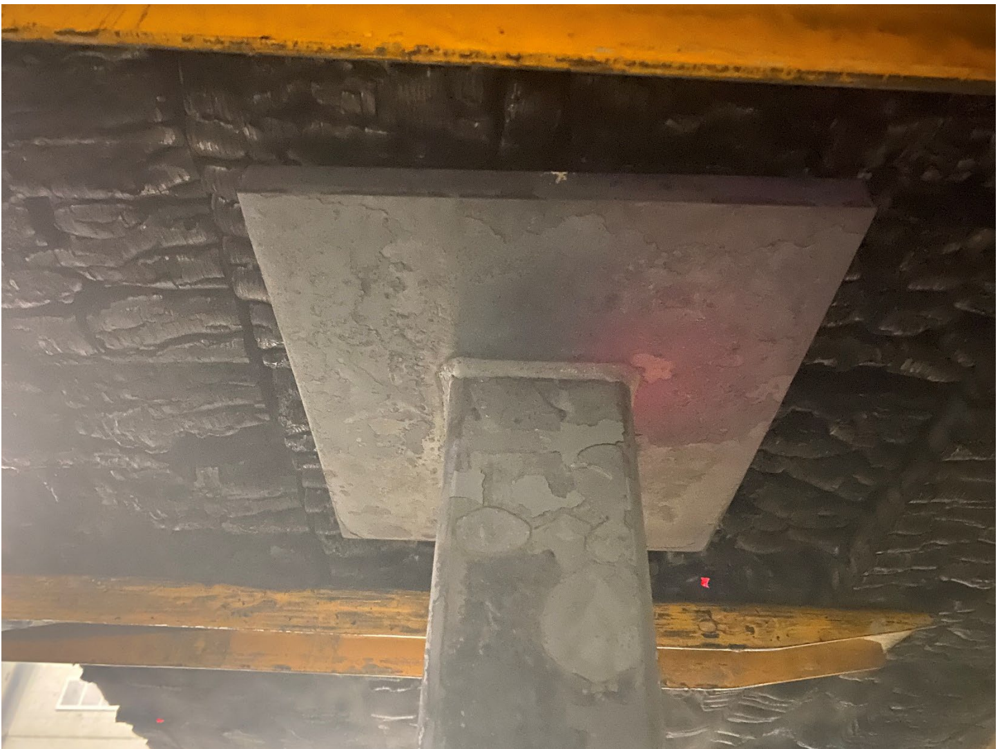
Figure 11. CLT floor / ceiling and steel column assembly post testing.
