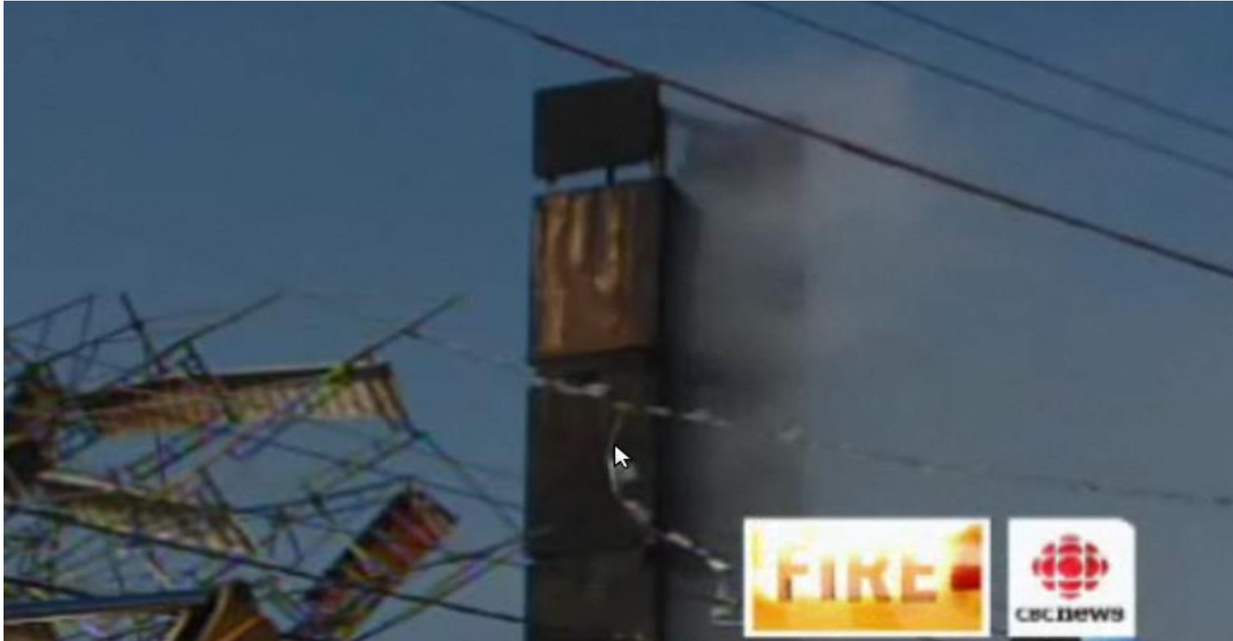
Laminated 2x6 elevator shaft
