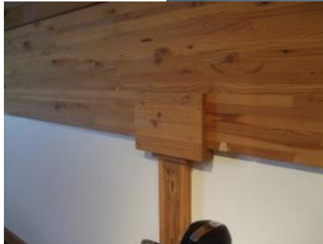
2h Fire Rated Connection The Landing, Vancouver
