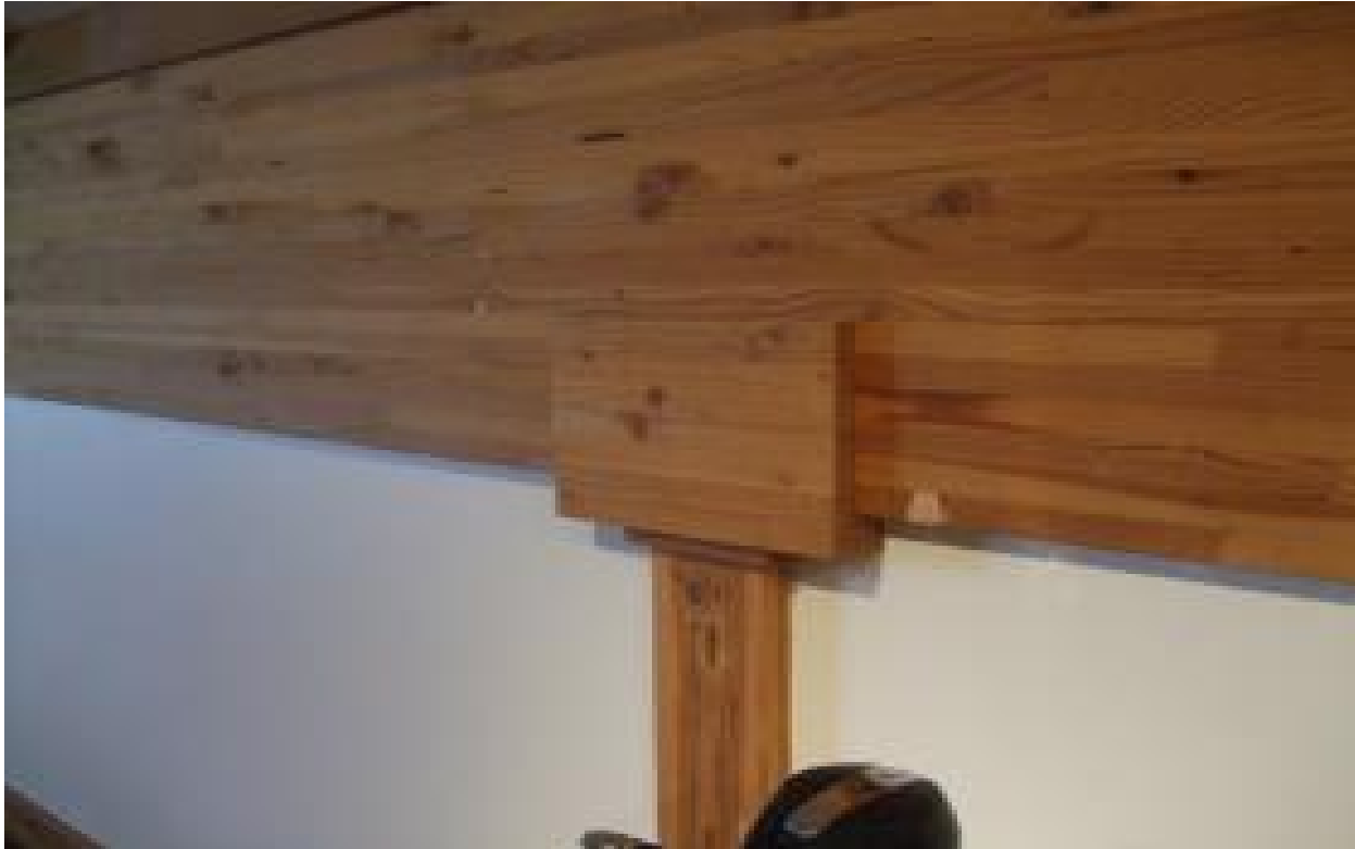
b) Connection covered with wood paneling
