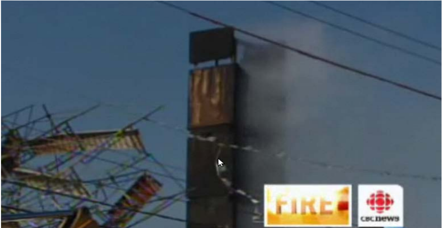
Laminated 2x6 elevator shaft
