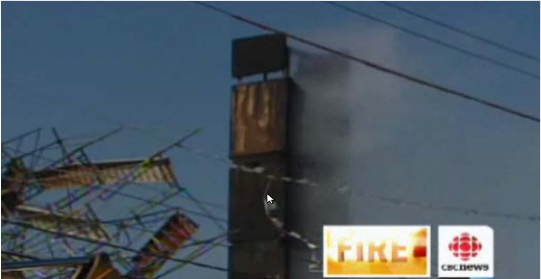
Laminated 2x6 elevator shaft
