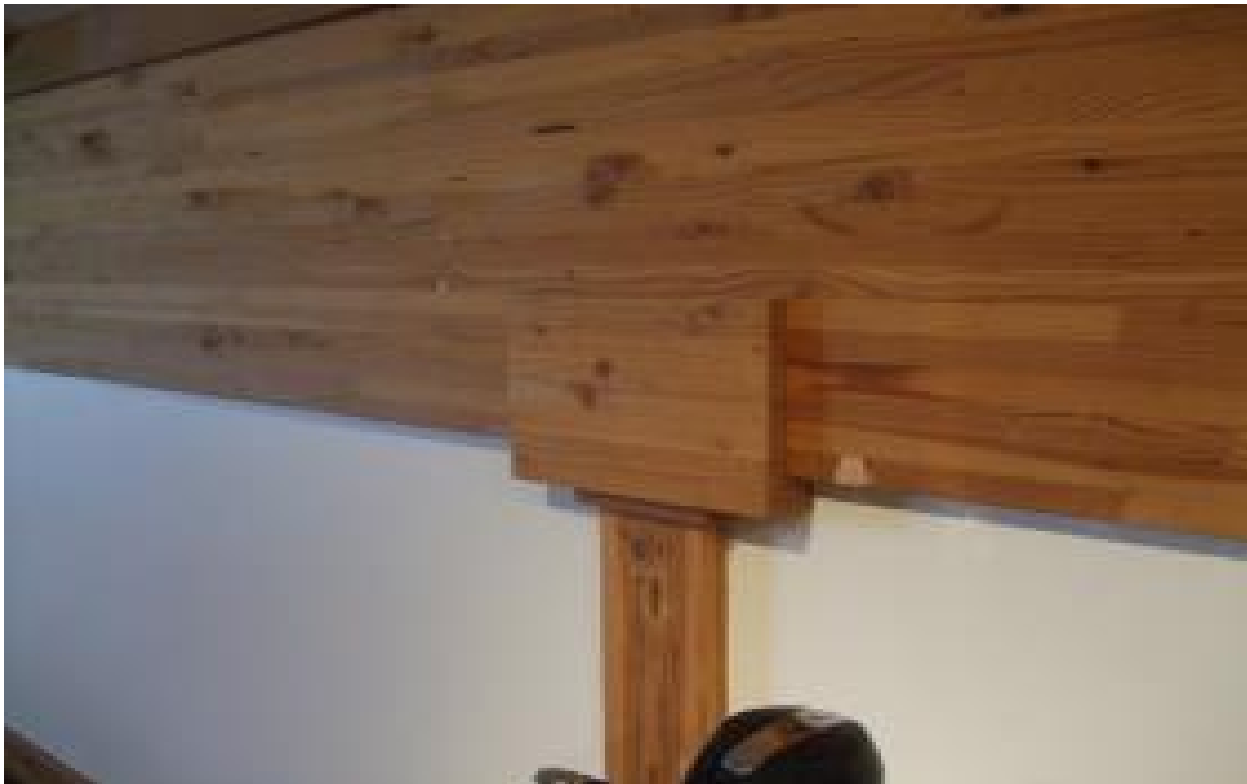
b) Connection covered with wood paneling
